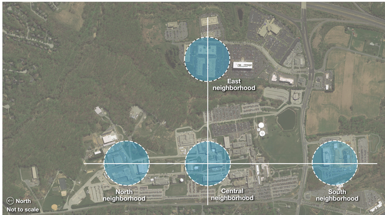
Figure 8. APL's campus neighborhoods. Application of the axial and nodal relationship diagrams reveals the four neighborhoods of the Laboratory's campus. This realization reframes the relationship between each area of the campus, recognizing the campus as an integrated community.
