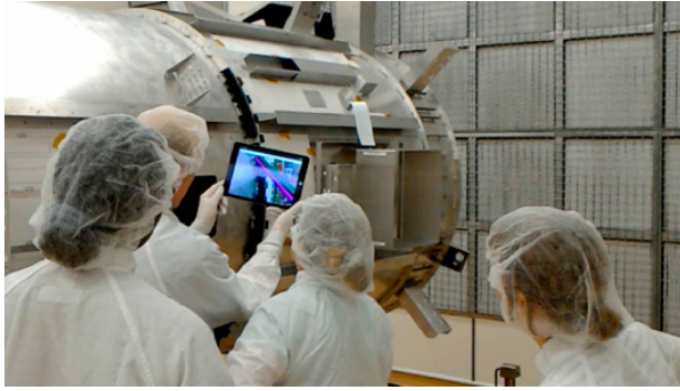
Figure 8. Prefabrication review using CAD model and AR tool. This photo shows engineers and fabrication technicians using Vuforia, with the CAD models superimposed on the physical fixture, to review the placement of the harness routing before the technicians begin to cut and place wire.
