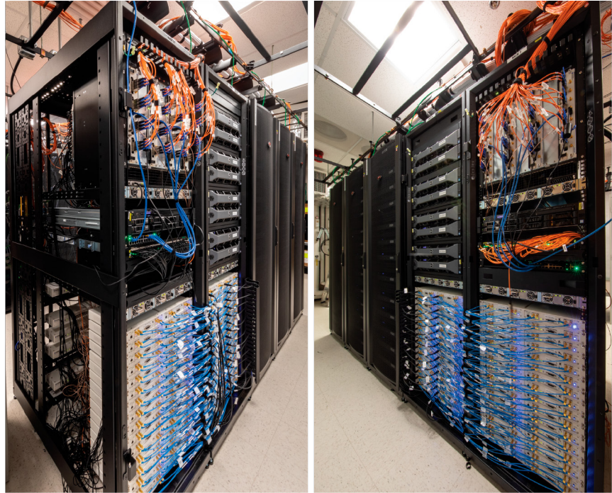
Figure 1. Photos of the Colosseum hosted in a server room on APL’s Laurel, Maryland, campus; it included 21 server racks comprising servers, SDRs, and network equipment. In October 2019 it moved to the Institute for the Wireless Internet of Things at Northeastern University.
