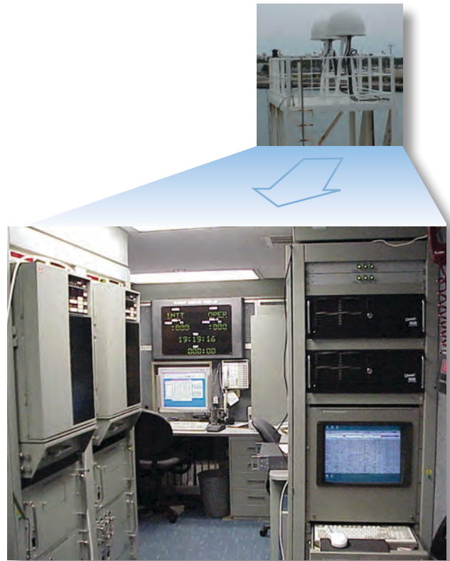
Figure 7. FTSS control van with ESHA antennas inset. The FTSS van contains telemetry and GPS tracking equipment. The ESHA antennas provide the S-band RF feed for these systems.
