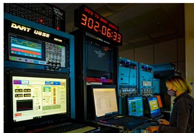
In the Ground System Equipment control room at APL, engineers perform tests and simulations on the DART spacecraft. (Credit: NASA/ Johns Hopkins APL)
